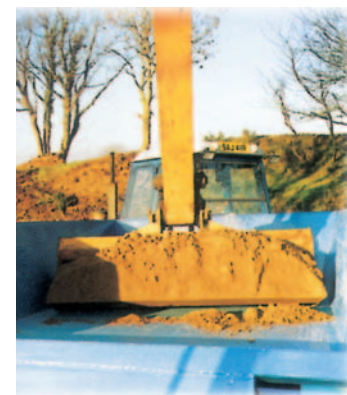
Easily scraped out with wide bucket
